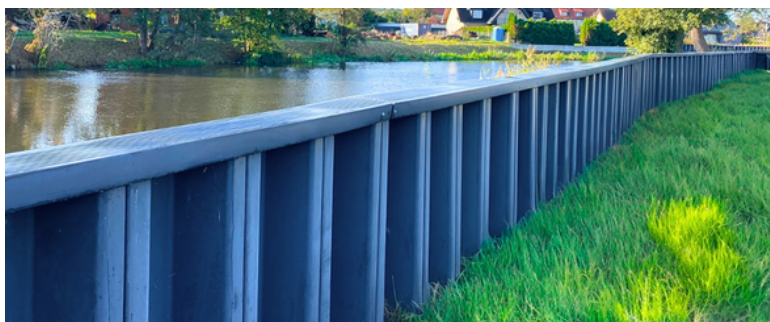
Sheet pile floodwall example
