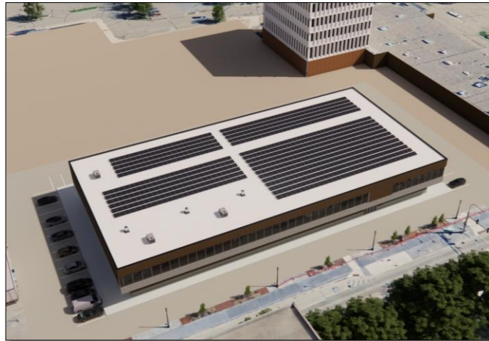
New Library ~239 kW Rooftop Solar Array
