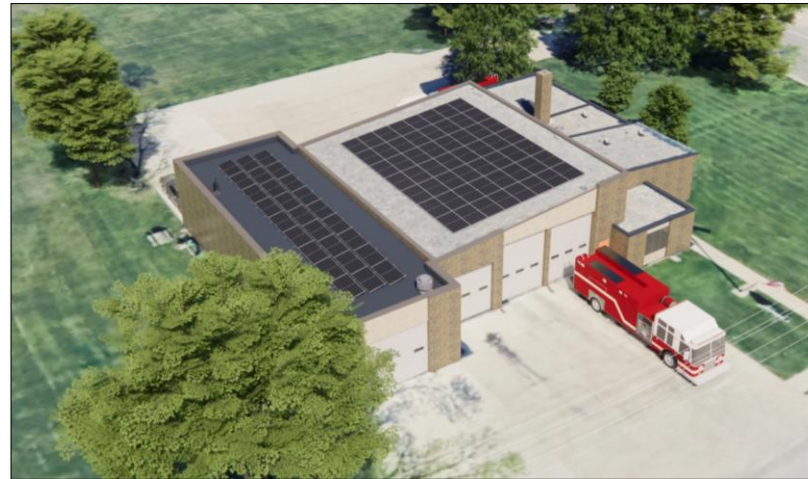
Fire Station #2 ~49 kW Rooftop Solar Array
