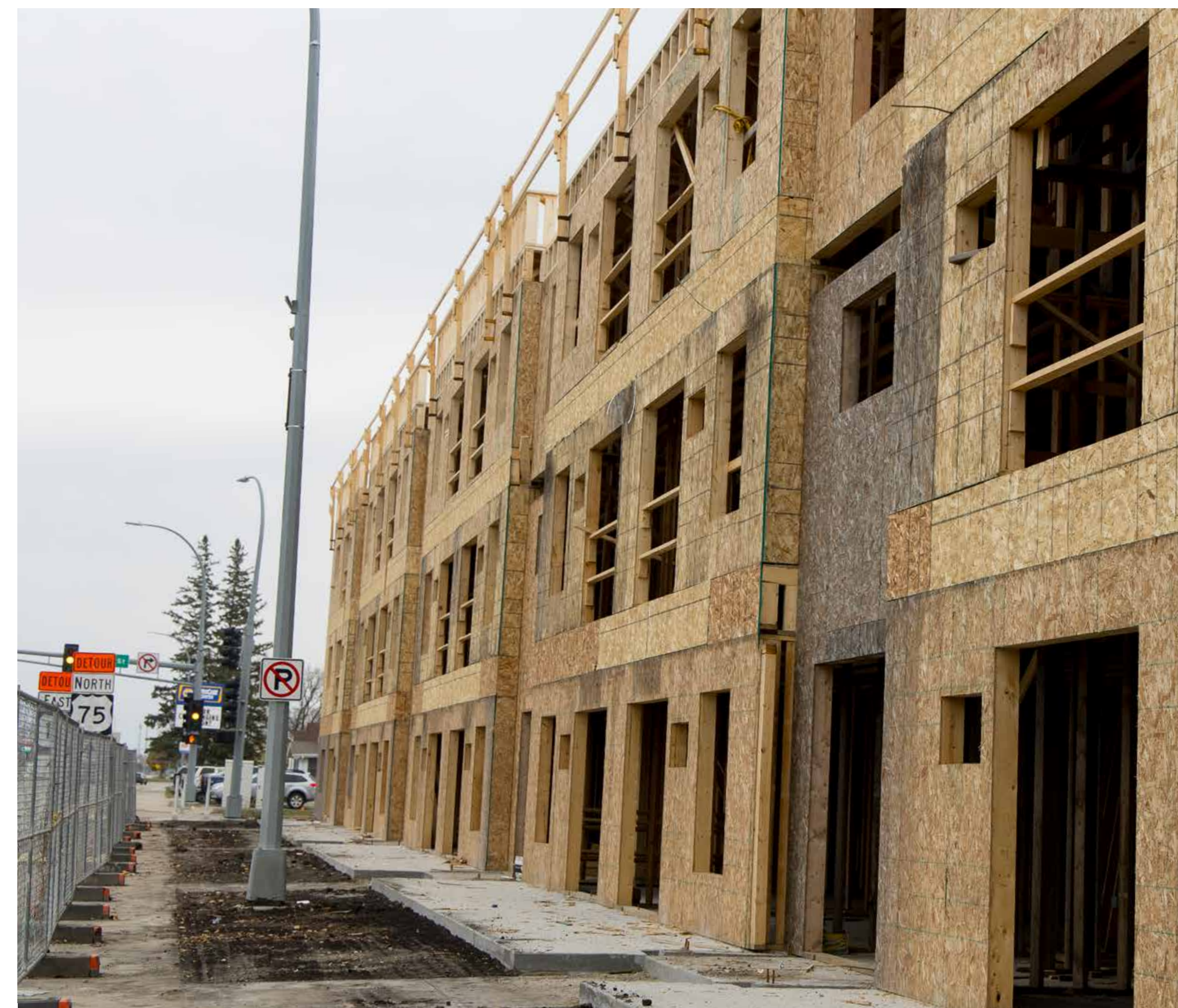
14th and Main Apartments
