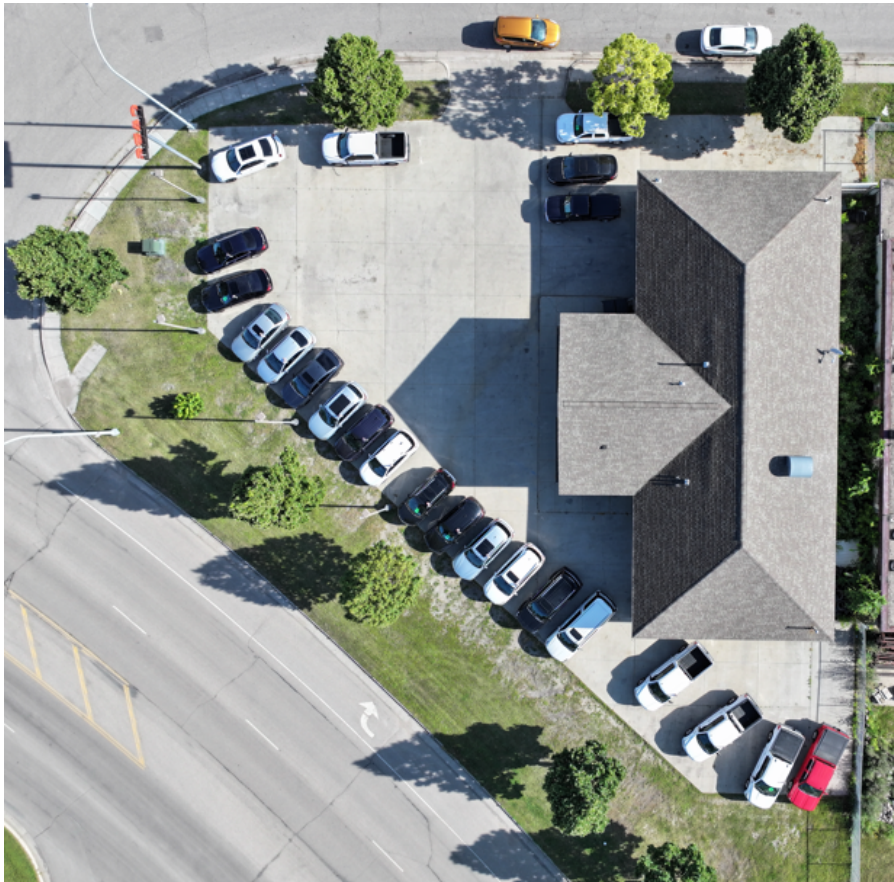
Aerial photo - July 17, 2025 Site parking - fully on hard surface lot
